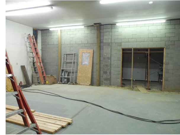
New block wall
