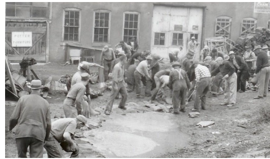
Back wall of the Megquier - Houck Building, 1956
