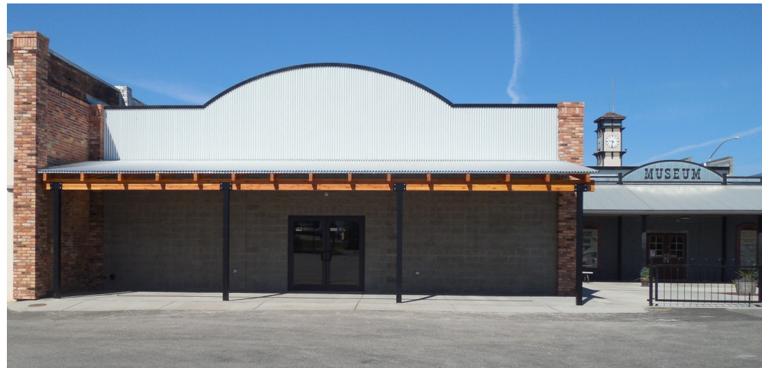
New Block Wall, 2016
